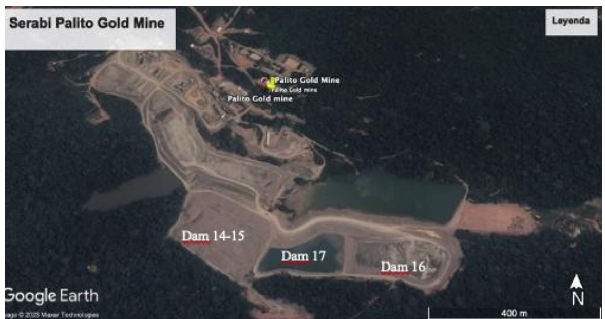
Figure 18-5: General View of Tailings Dam Area
