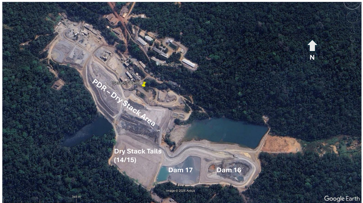
Figure 18-5: General View of Tailings Dam Area
